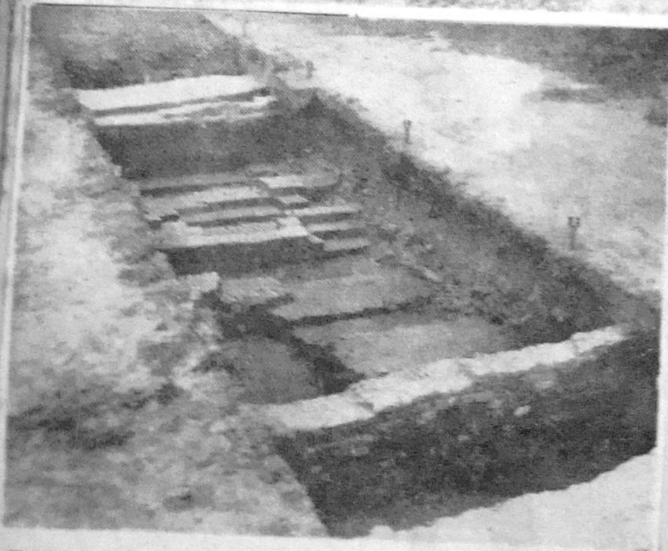
EARLY BRICKMAKING AT JAMESTOWN —Top picture shows detailed construction of kiln. The bricks in herringbone pattern are ready for firing. Note the partially fired brick and tile lying inside the firing chamber to the left. Bottom picture shows a completely excavated 10-foot section of brick and tile kiln. Four of the five firing chambers can be seen in the photograph. Here the first bricks made in the colony were manufactured. These and many other interesting relics of early colonial activity have been uncovered by the United States Park Service.
